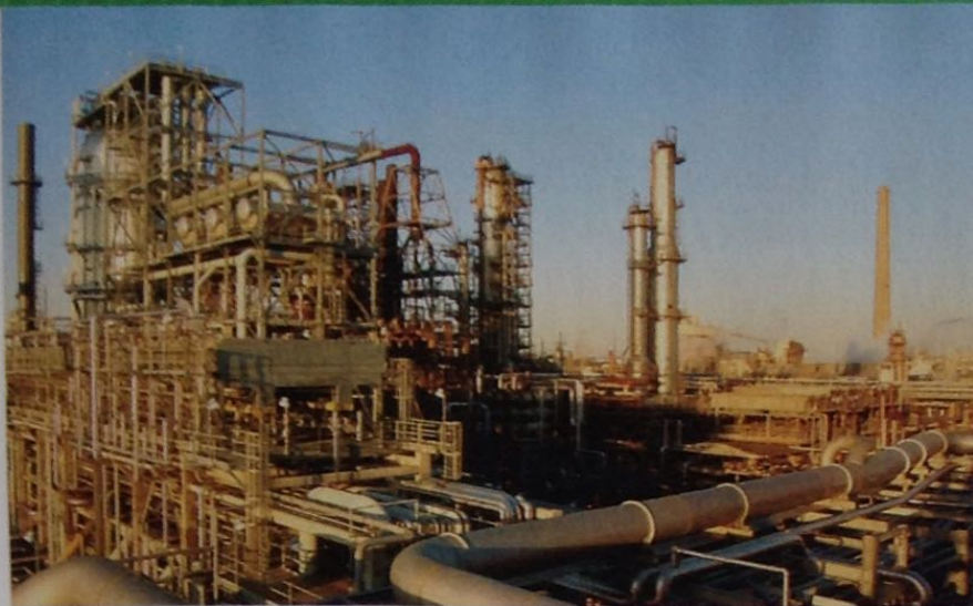
Figure 2 Some refineries use a process called distillation to separate petroleum into various types of petroleum products.
